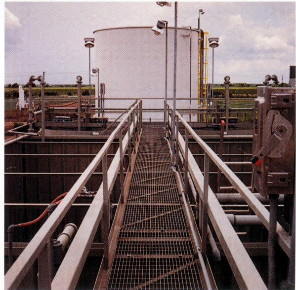
The Field-Erected ADDIGEST model configurations include both circular clarifiers (seen above) or hopper clarifiers.
