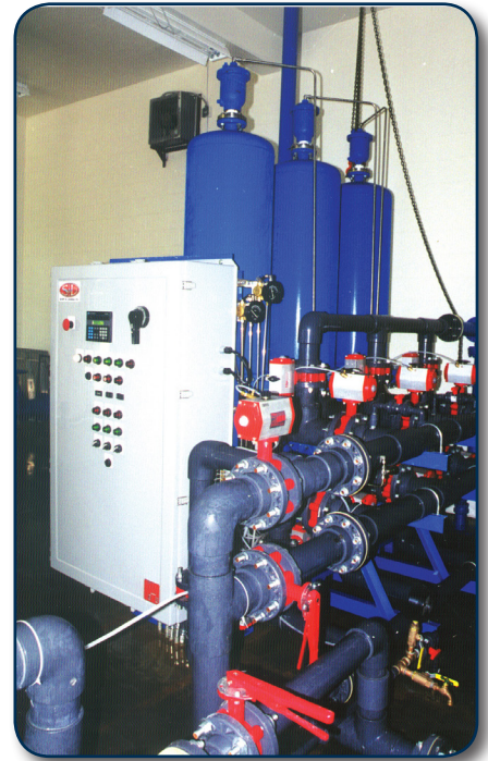
For even larger flows, AX50 units are manifolded together
