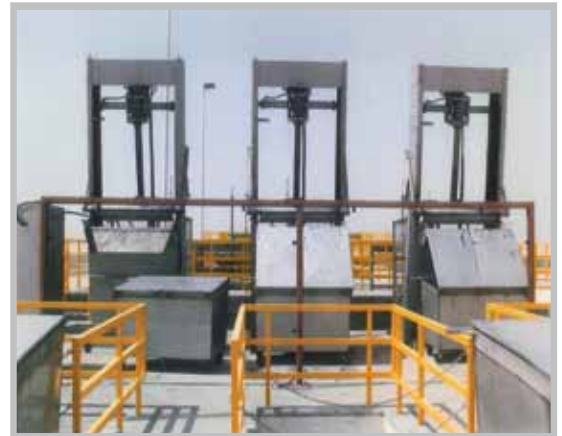
Above: Vertical Mark CI™ with full enclosure discharging into a Schloss™ Hydraulic Ram Press. At right: Three Mark CI™ Screens serve a large plant in the Middle East.
