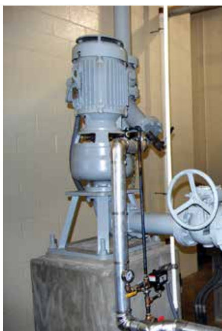
Remote-mounted, Flooded Suction Turbo Grit Pump
